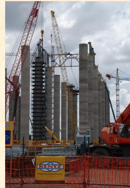
Medupi Power Station
