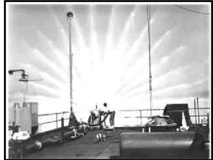
Water flow test of pintle injector for Air Force 250,000 lbf Engine
